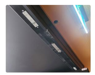
The YD30S has a high holding force, in excess of 1000kg, and release under sideload pressure of up to 600kg.
